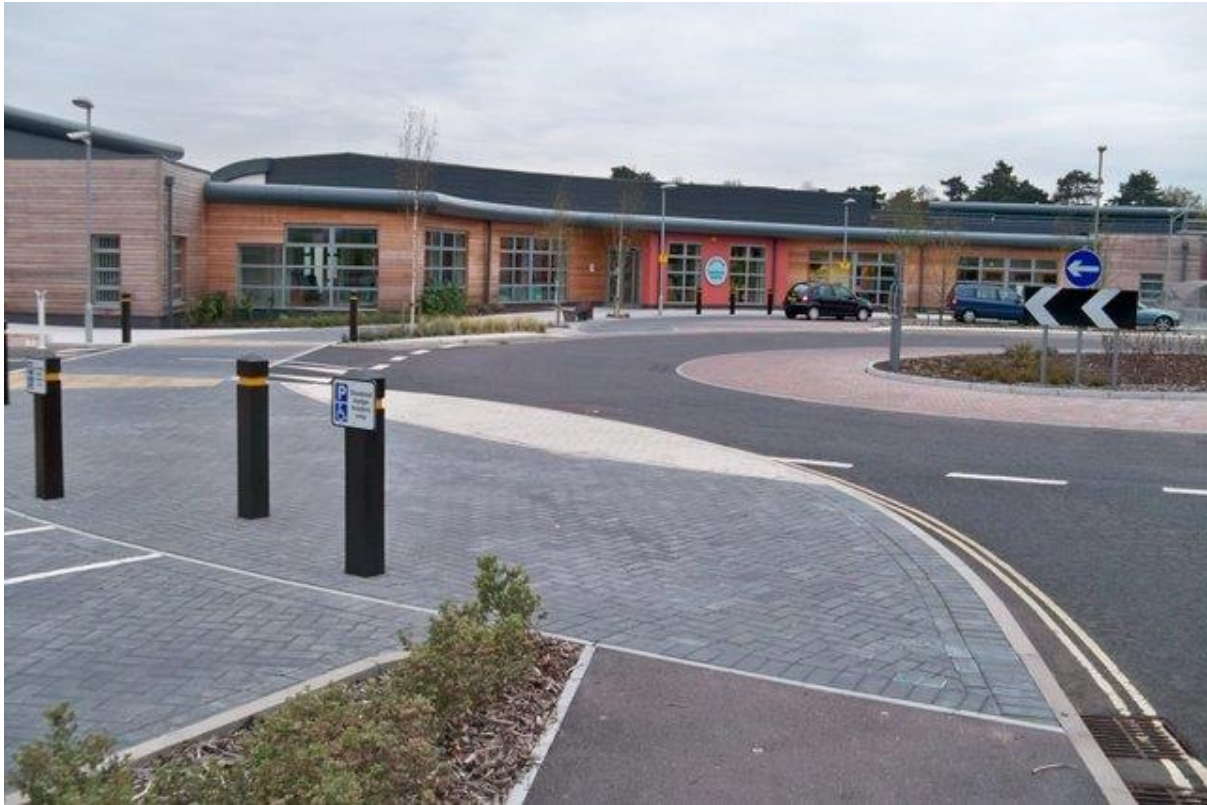
Figure 9 - Fareham Community Hospital
